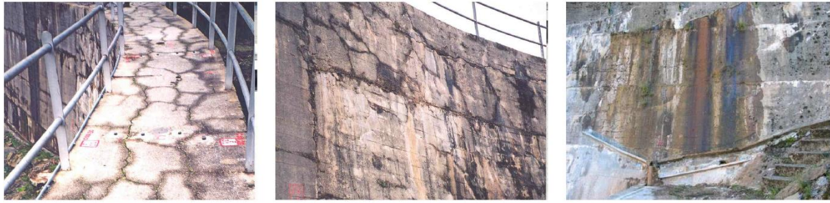
Fig. 15 – Alto Ceira dam. Cracking patterns on the crest and on the downstream surface, and device to measure the leakage through the dam’s body (Custódio et al., 2020).
