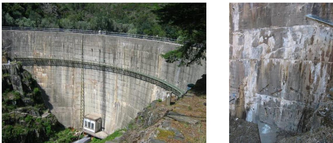
Figure 12 - Alto Ceira dam. General view and detail with extensive cracking and exudation (COST TU1402: Quantifying the Value of Structural Health Monitoring).
