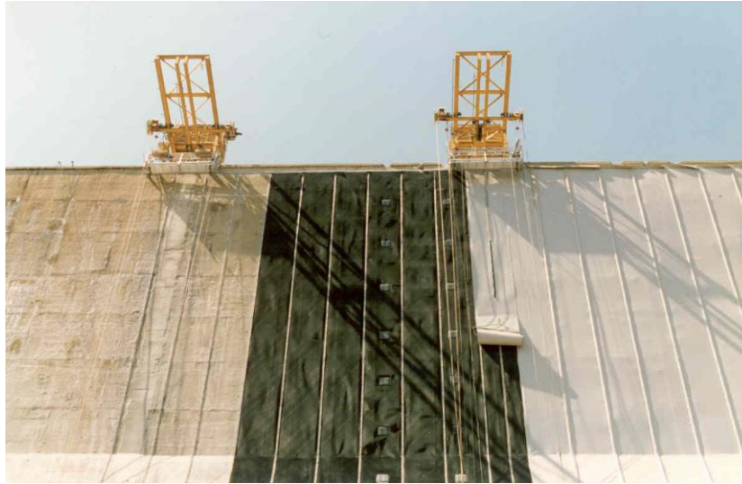
Figure 24 – Pracana dam. Stage of installation of the upstream impervious membrane (Batista, 2022).
