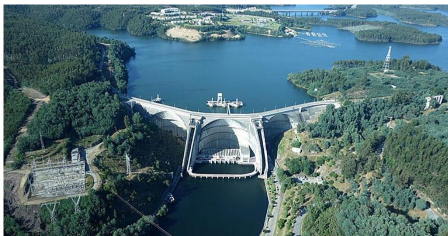
Figure 5 - Aguieira dam and image of part of the reservoir showing one of the seven bridges.
