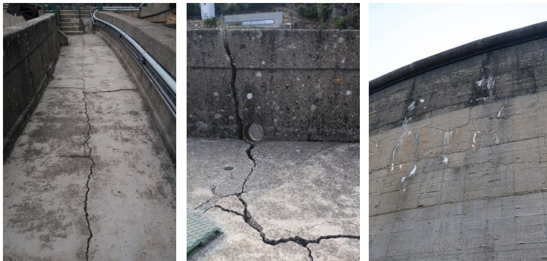
Figure 19 – Santa Luzia dam. Results of crack survey of upstream surface due in October 1998 (Piteira-Gomes et al., 2022a; Batista, 2022).
