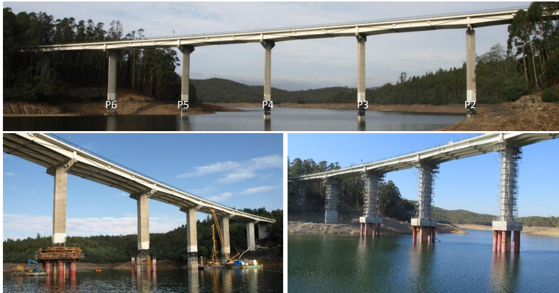
Figure 8 - Criz II bridge before and at during the rehabilitation works (Santos et al., 2022).
