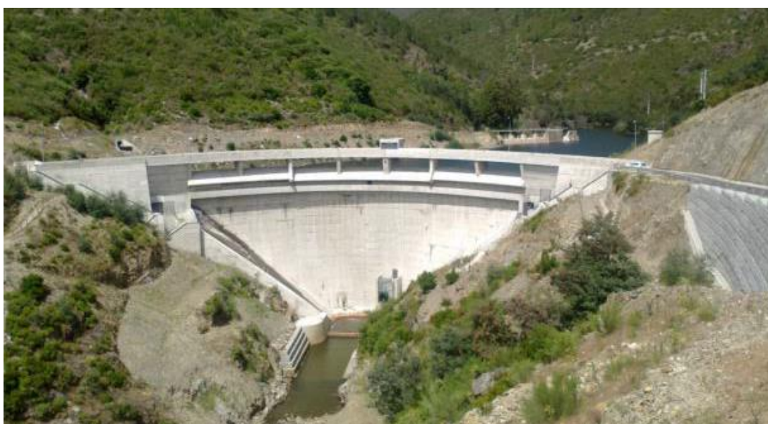
Figure 17 – The new Alto Ceira dam (Leitão et al., 2015).
