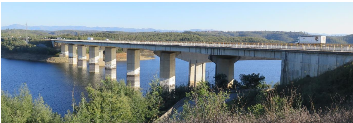
Figure 7 – Foz do Dão bridges: the old bridge in the foreground and the new bridge behind.
