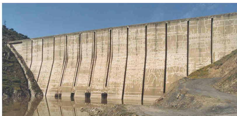
Figure 23 – Pracana dam. Map cracking of the downstream and upstream faces.
